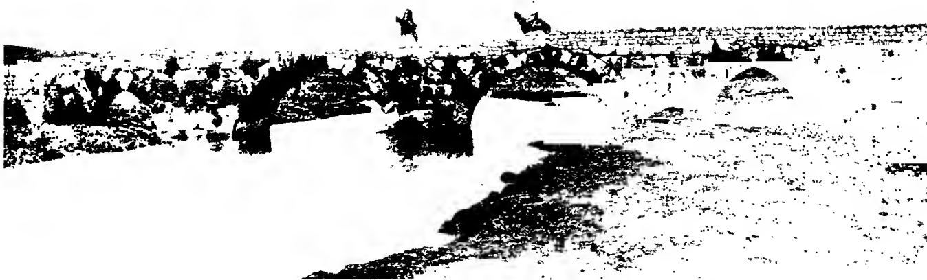
Djîsr il-Madjdal, ancient Roman bridge on the road between Hamā and Apamea, about two hours and a half north of the former. The arches are each about 6 m. broad, and the roadway is 5.60 m. wide.
